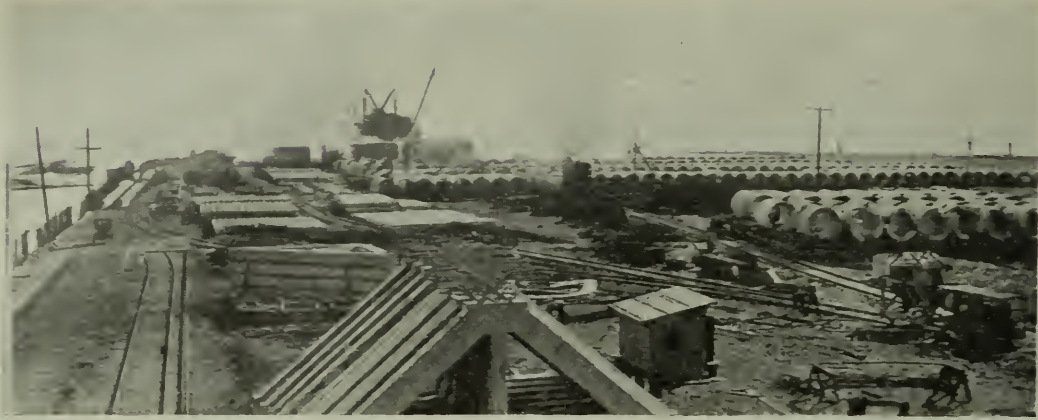
CASTING YARD FOR PRE-CAST UNITS.
